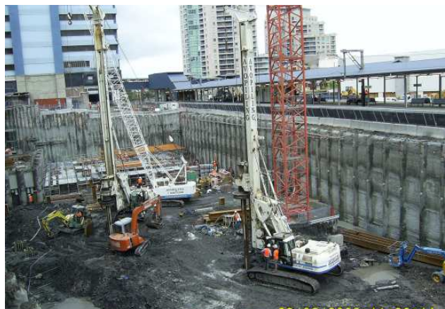
Exposed contiguous Piles and progress of Foundation piling
