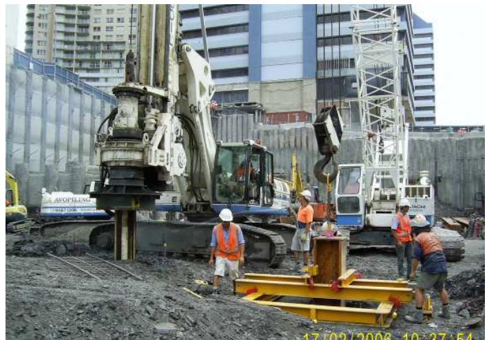
Guide frame set up ready to cast pile with embedded welded column
