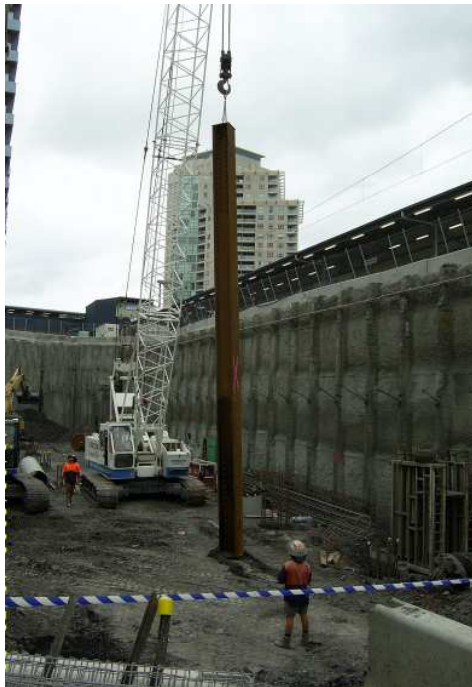
Lifting welded column into place
