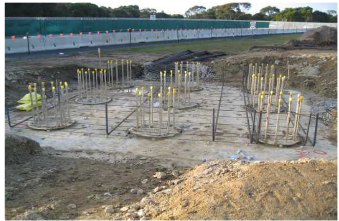
Column Reinforcement installed and cast with bored piles
