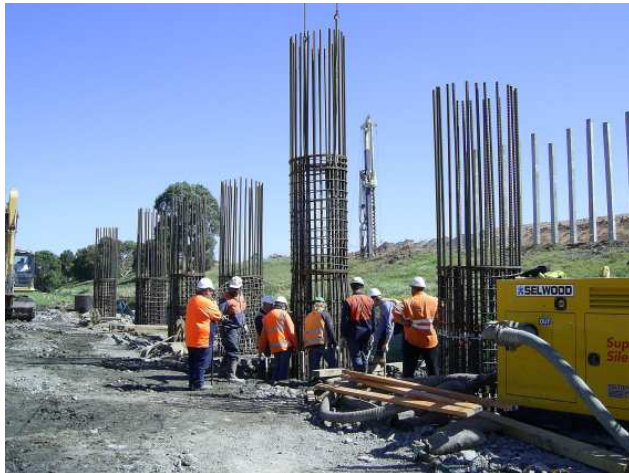
Column Reinforcement installed and cast with bored piles
