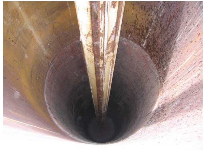
Retaining Wall – 13- contiguous Piles 900mm & 1200mm dia.
