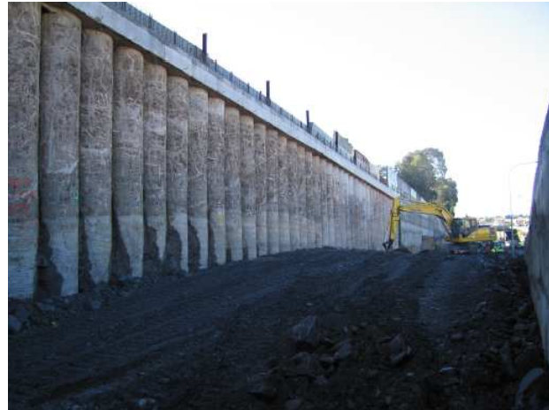
Retaining Wall – 13- contiguous Piles 900mm & 1200mm dia.
