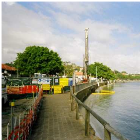
Drilling with environmental controls in place
