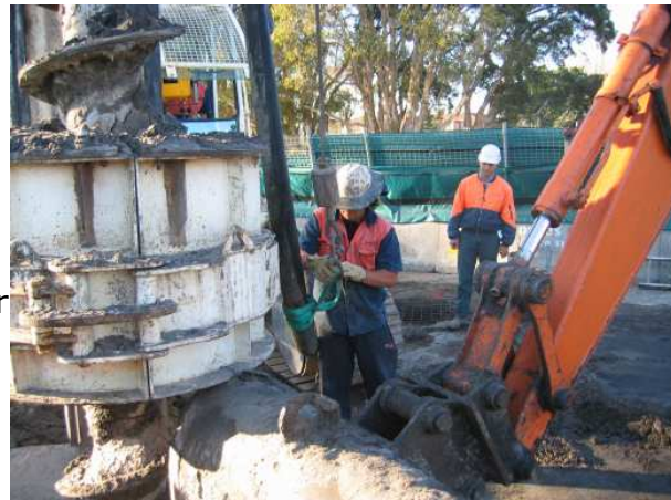
Managing the drilling process
